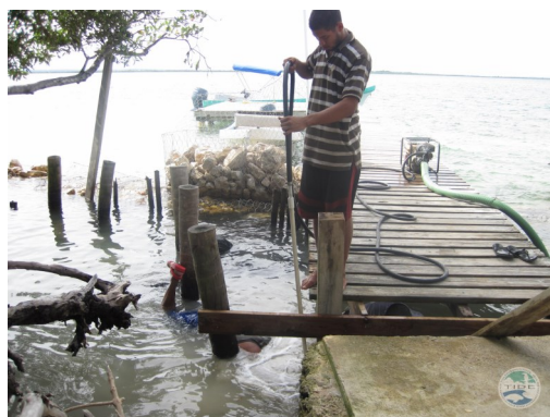
Repairs to the dock at Abalone Caye
