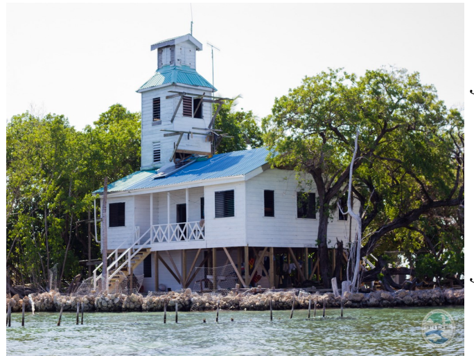
The newly restored Abalone Caye
