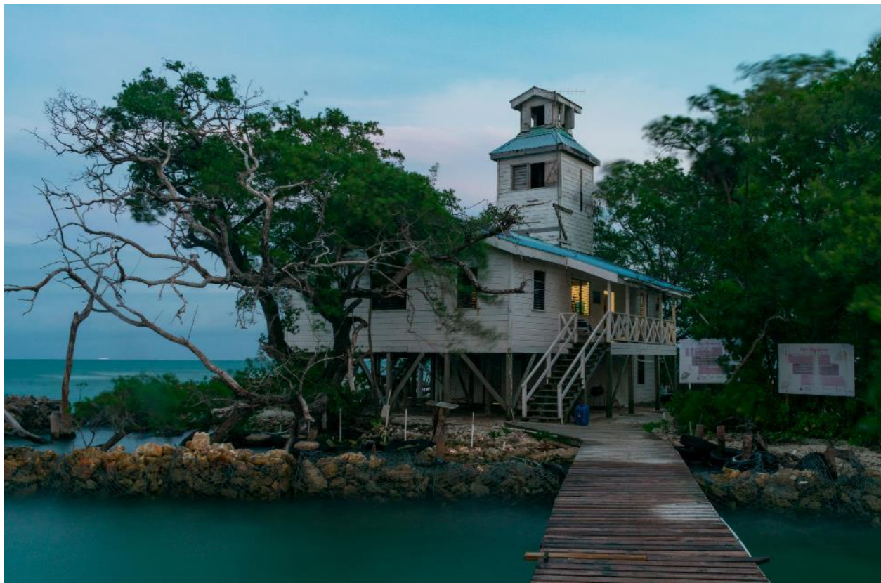
Picture 2: Showing Abalone Ranger station before renovations
