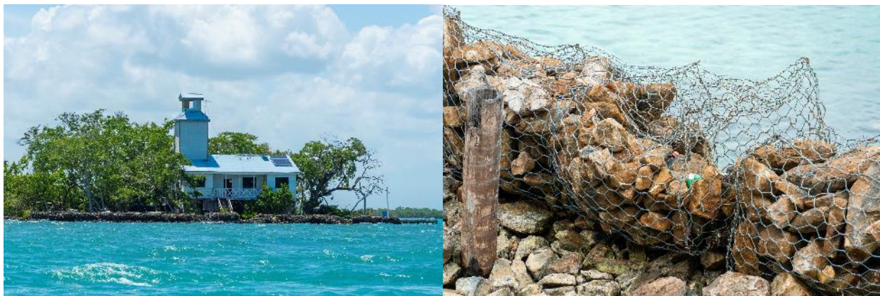
Figure 11: Showing Abalone Caye and the seawall Seawall out at Abalone Caye
