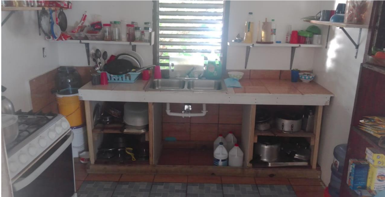
Figure 9: Refurbished kitchen with tile countertop and floor
