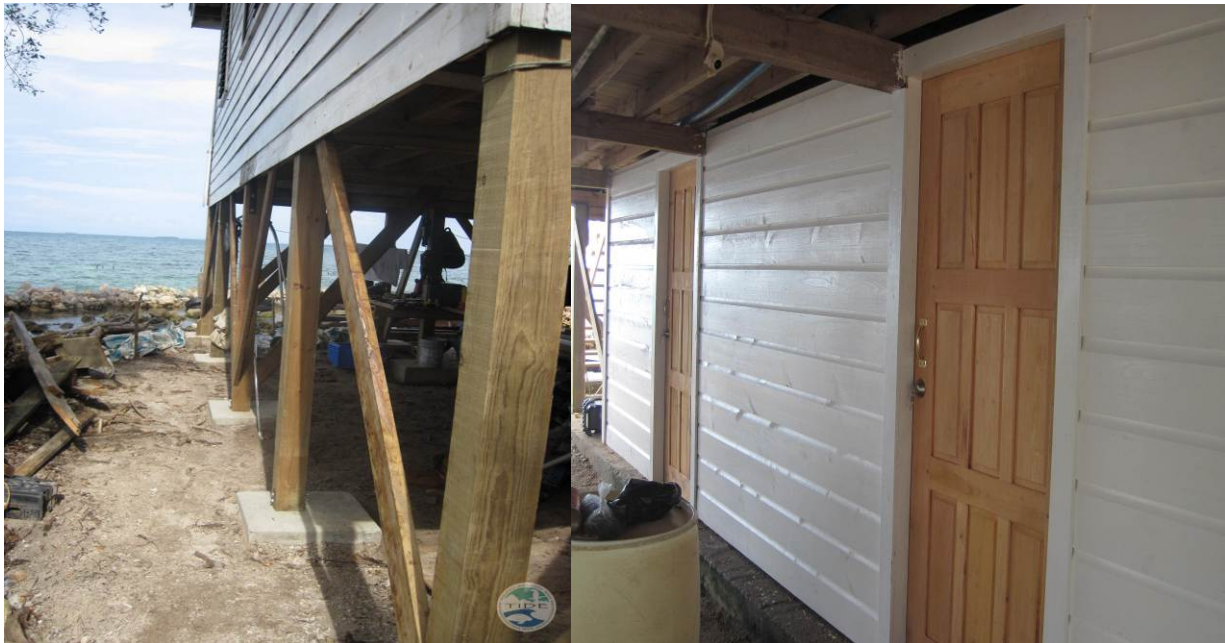
New hard wood posts and cement footings
