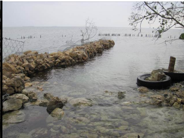
Gabion baskets filled with rocks lining the coast of Abalone Caye
