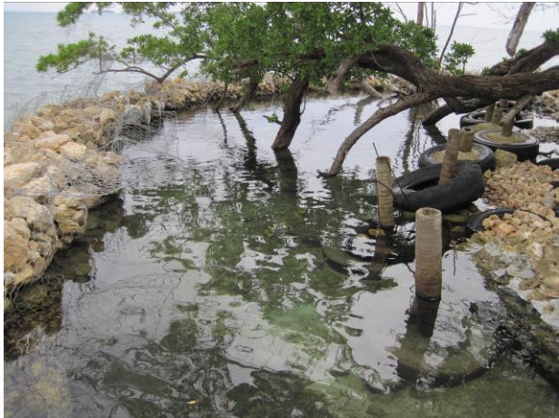
Gabion baskets filled with rocks lining the coast of Abalone Caye
