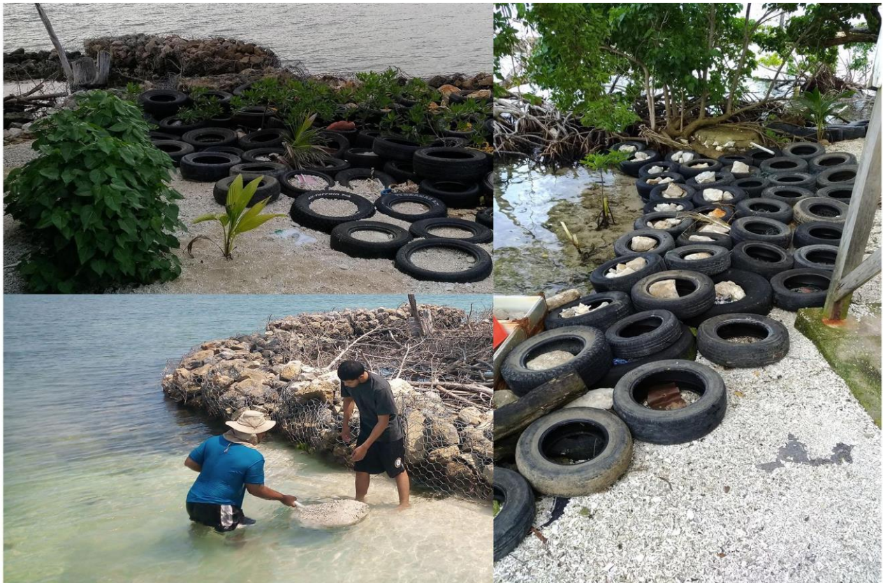
Figure 11: Erosion control done around Abalone Caye
