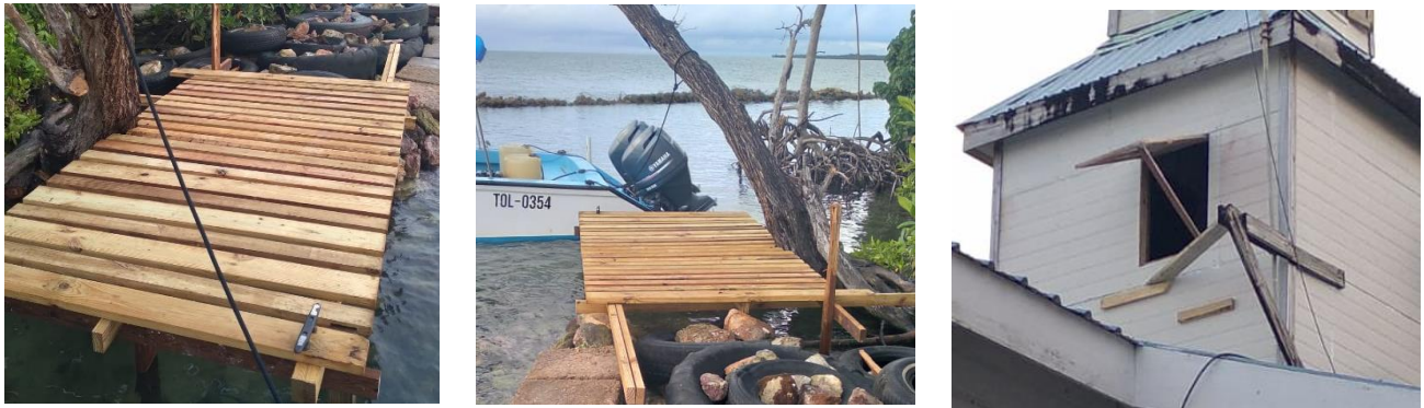
Figure 8: Showing infrastructure maintenance done at Abalone Caye
