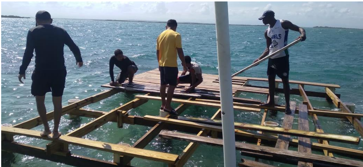
Figure 12: Rangers and the Belize Coast Guard personnel working to refurbish the Dock.
